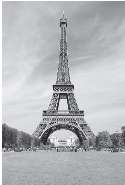
Figure 1.2 Two legs of the Eiffel Tower are underlain by softer soils, and thus could have settled more than the other two. Fortunately, Eiffel carefully explored the soil's conditions, recognized this potential problem, and designed the foundations to accommodate these soil conditions. His foresight and diligence resulted in a well-designed foundation system that has not settled excessively (Courtesy by Shutterstock).
