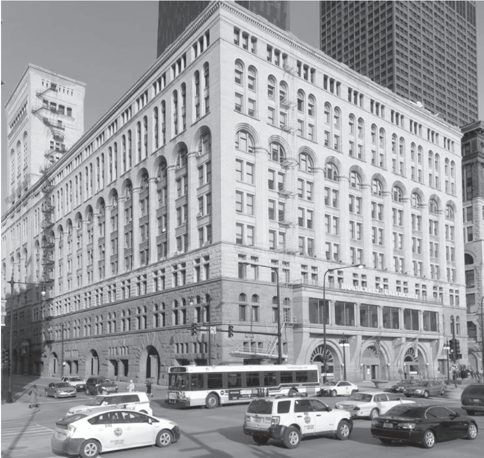
Figure 1.3 The auditorium building in Chicago experienced 28 in of settlement, but is still in service more than a century after its completion. This structure helped usher in new foundation designs that are less susceptible to settlement.
